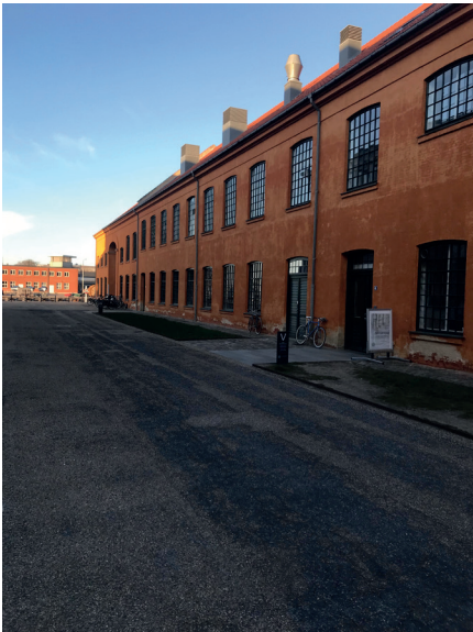
University building with a huge printing workshop.
